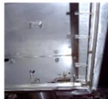
3/16 Thick Steel Flat Bar 19 Inches Long And 1 1/2 Inches Wide
